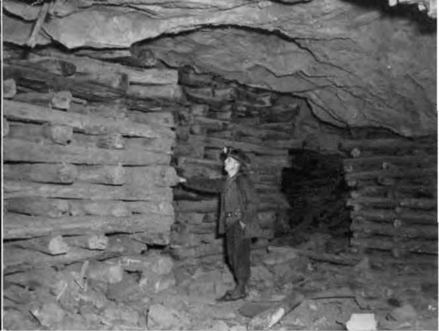
Leonard Lapointe checks cribbing between E Stope and Pillar.
