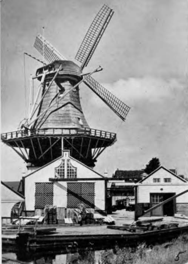
This windmill operates a sawmill.
