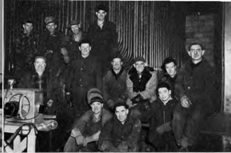
Machine shop crew at work on Fuming Plant Boilers.
