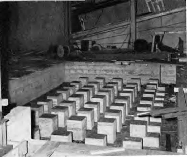
Foundations for electric furnace.
