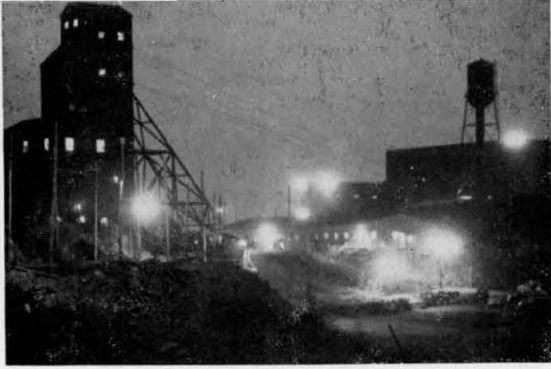
South Main Shaft by night.
