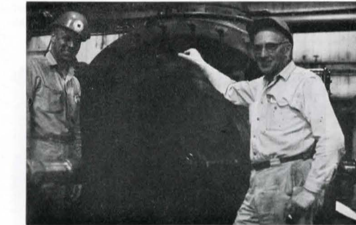
Ray Mullaney and Forbes Duncan have the old '981' down for repair.
