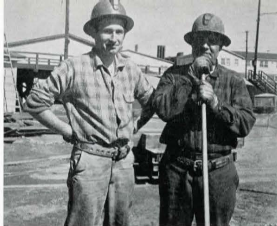
Bryant McFarlane and Paul Petrychko cleaning up around north main shaft.
