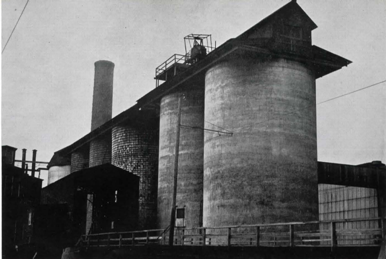
Smelter coal bins.
