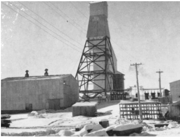
Chisel Lake hoist house and production shaft at left.
