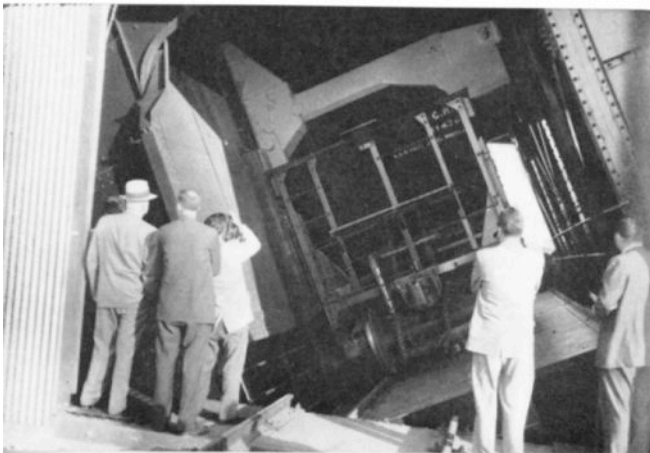
First car of ore from Chisel, September 2, 1960, locked in the tippie at Flin Flon, on its way to being turned over and cleared of ore.
