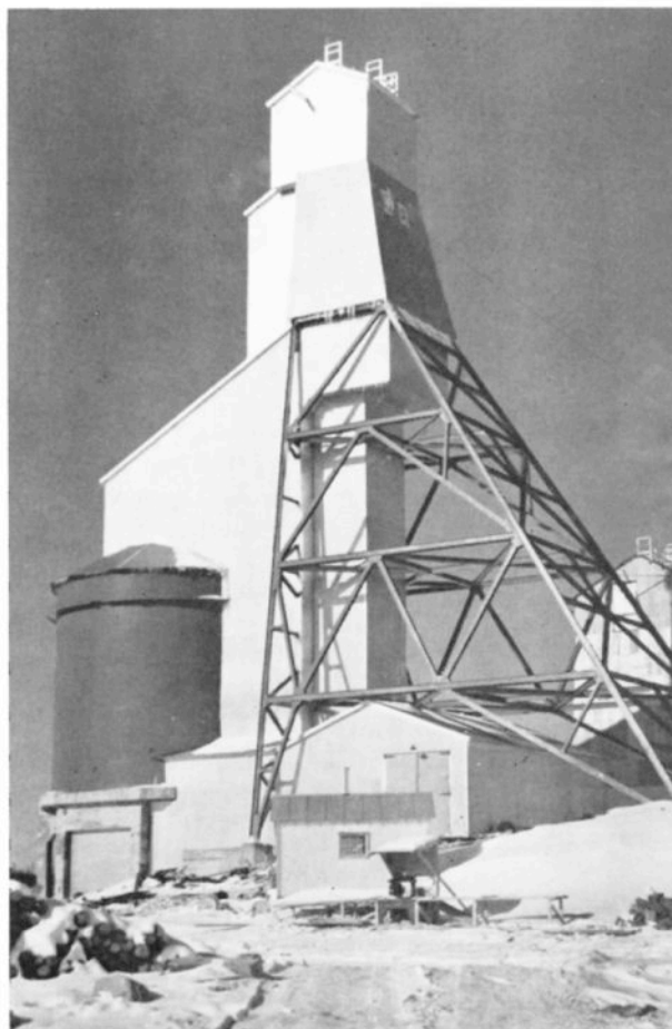
Headframe for Chisel Lake Mine, first property to be brought into production in the Company's Snow Lake field.
