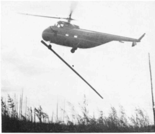
Toting power poles to speed up power line construction.
