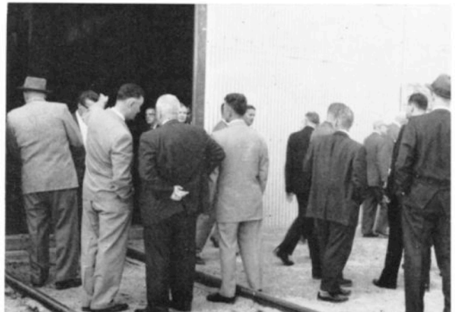
Company president, then General Manager, Eric Austin, second from left, explaining to a guest what happens to the ore after it is dumped from car.
