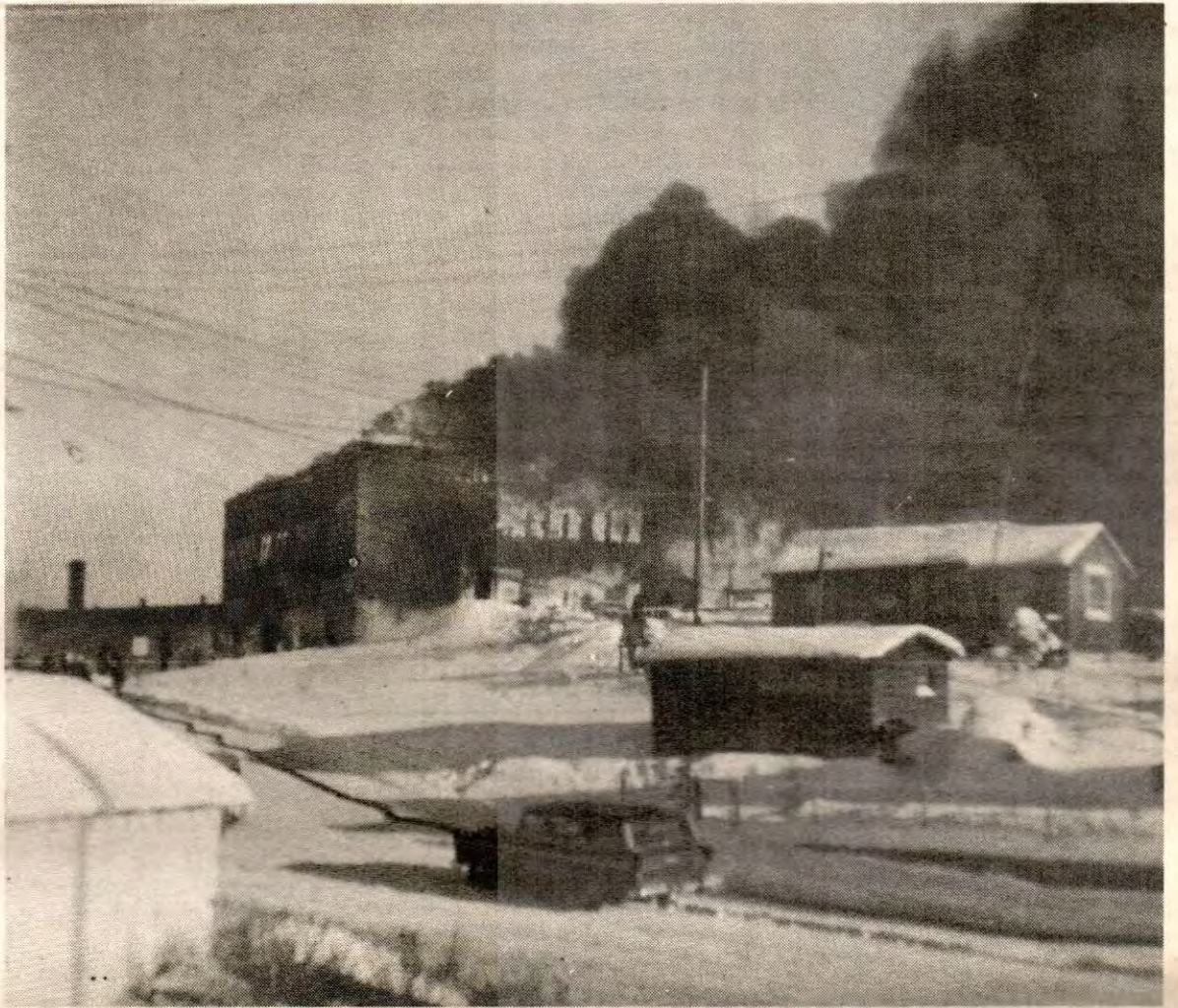
Flames leap into the air as Terrace School burns.
