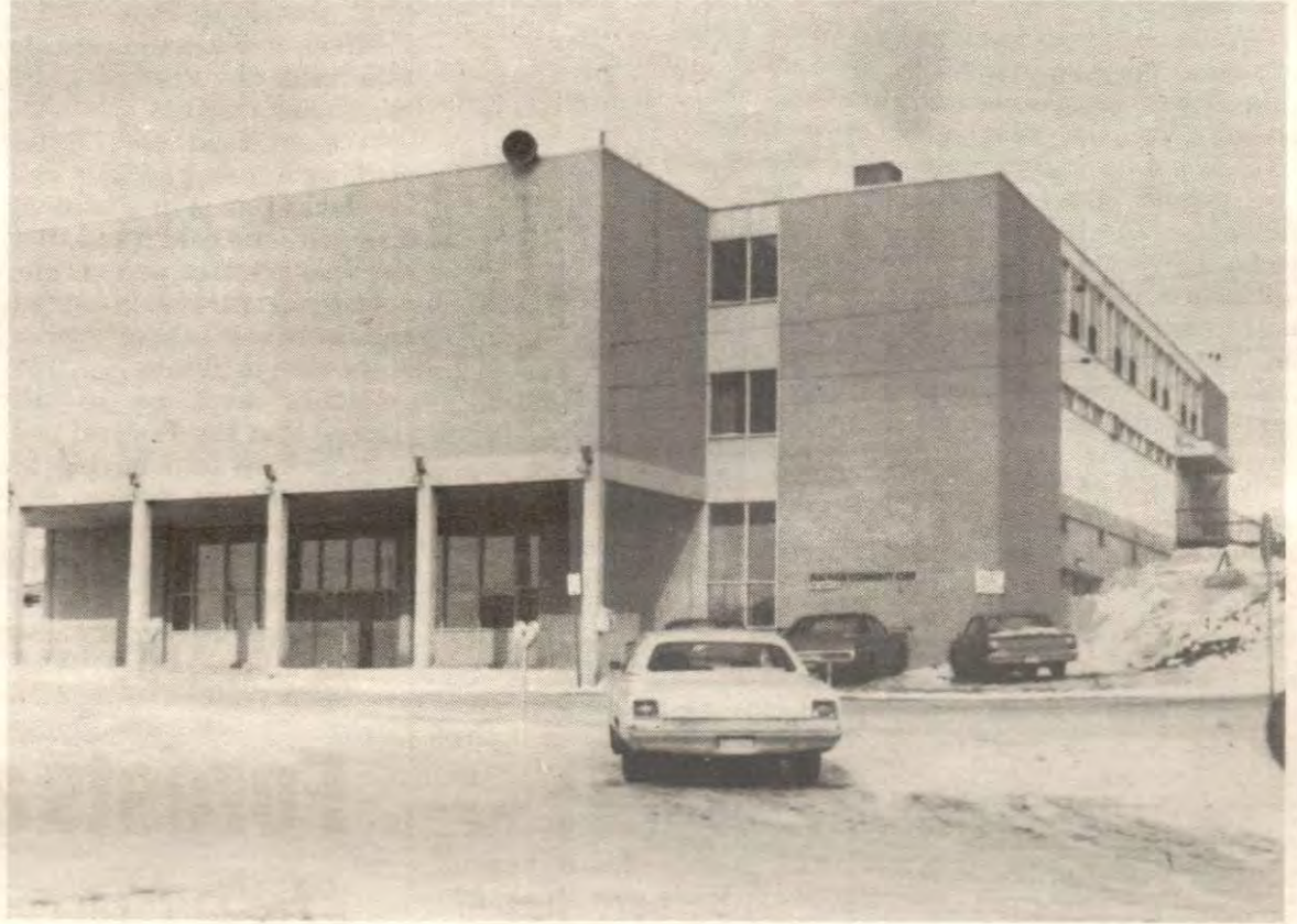
The Flin Flon Community Hall following its completion.
