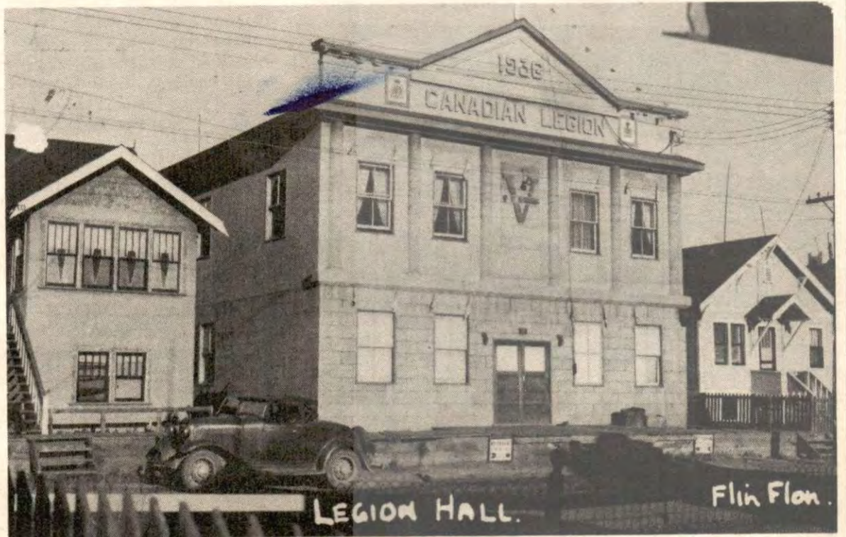
Picture 1 - Legion Hall at 73 Hapnot Street during the war years.
