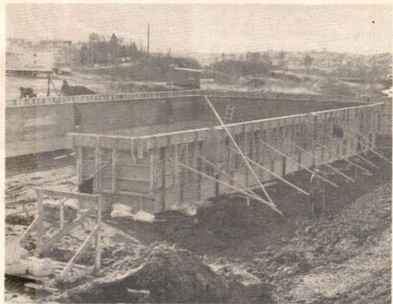
Aqua Centre under construction.
