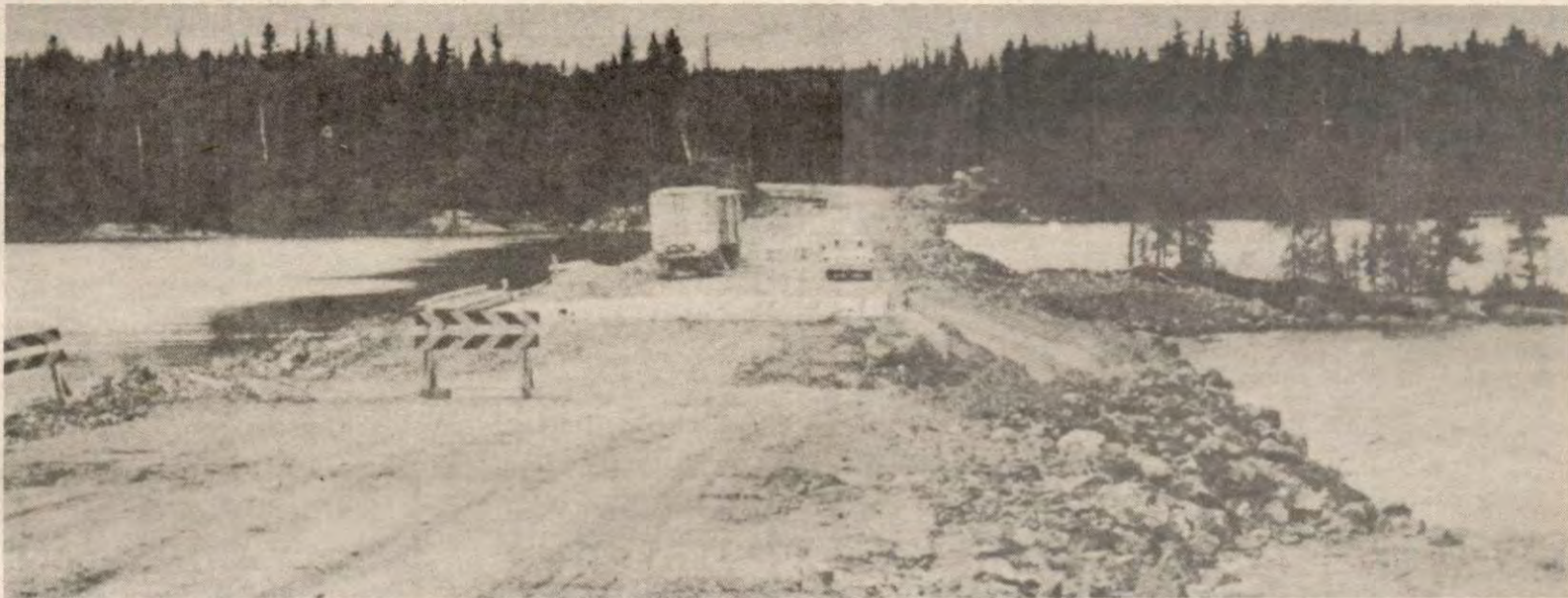
Building the bridge along the Schist Lake Causeway.
