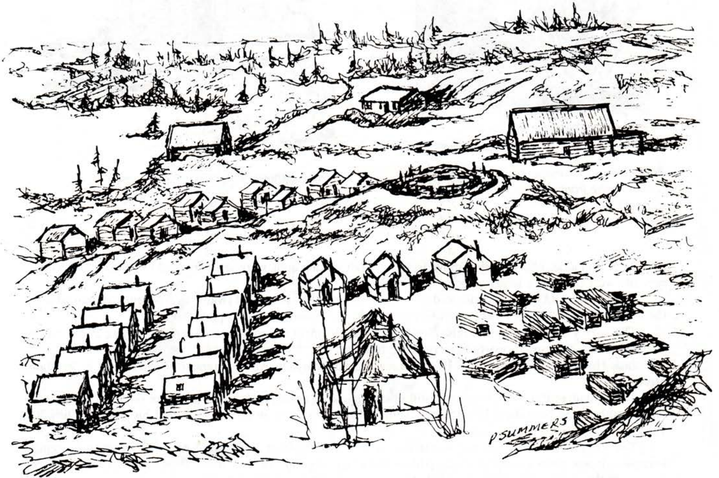
The sinking of the North Main Shaft (centre) with Hone's Store to the right. Tents housed the construction workers. Flin Flon Lake can be seen at the extreme left. 1929
