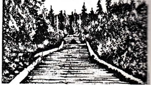
Corduroy road between Ross Lake and Flin Flon. Photograph taken from the 1935 issue of the C.I.M.M., paper by R. E. Phelan on 'History of Flin Flon Mine up to Construction'.
