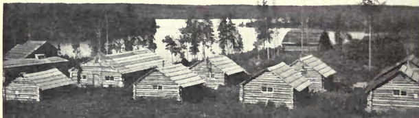
Camp Buildings on Flin Flon Property
