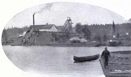
Mandy Mining Company's Plant at Schist Lake, showing Power House, Head Frame, Barges, Etc.
