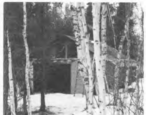
Lost Haven Cabin under construction.
