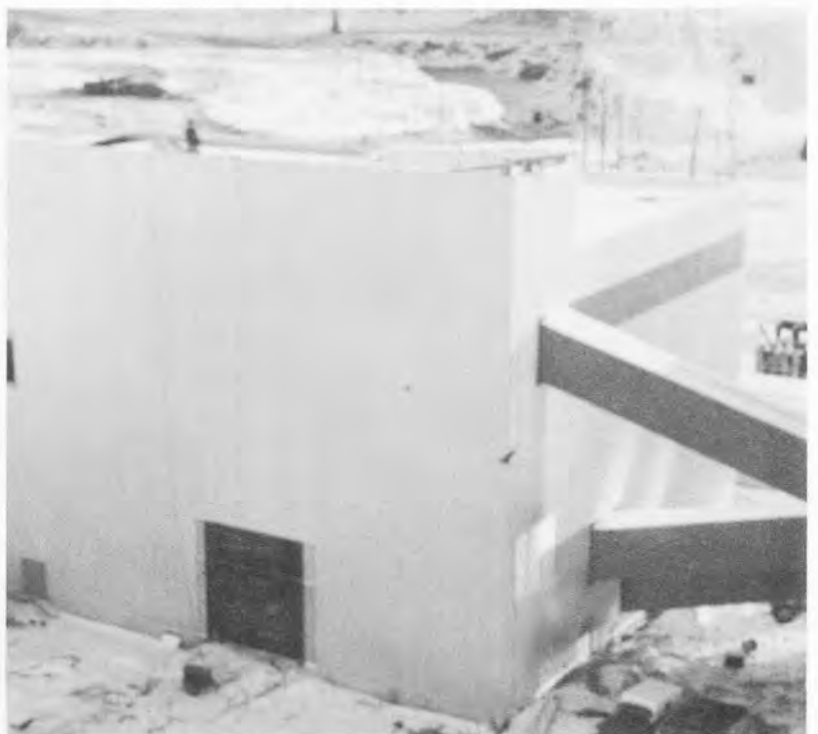
Secondary crusher, November 1972
