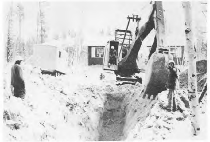
Installing Hydro Lines
