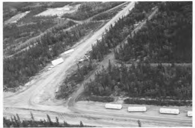
Construction Trailers being positioned 1971
