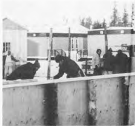
Constructing outdoor rink
