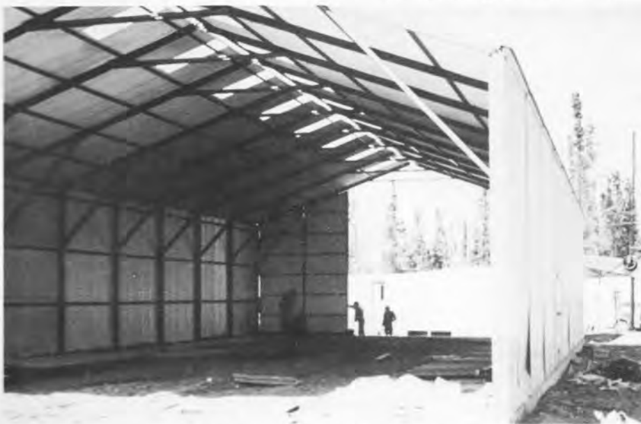
First recreation hall being built.
