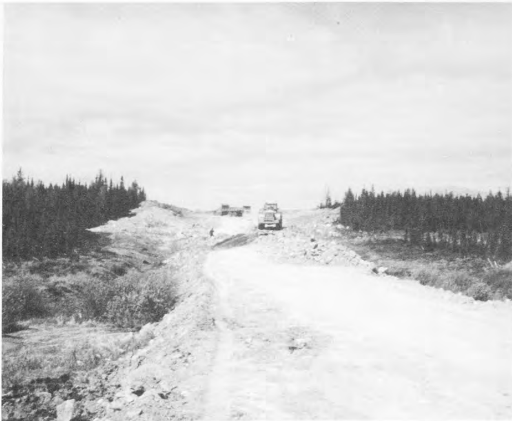
Road link to Thompson
