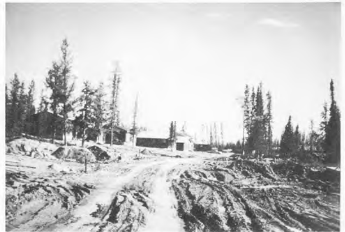
Partially completed homes
