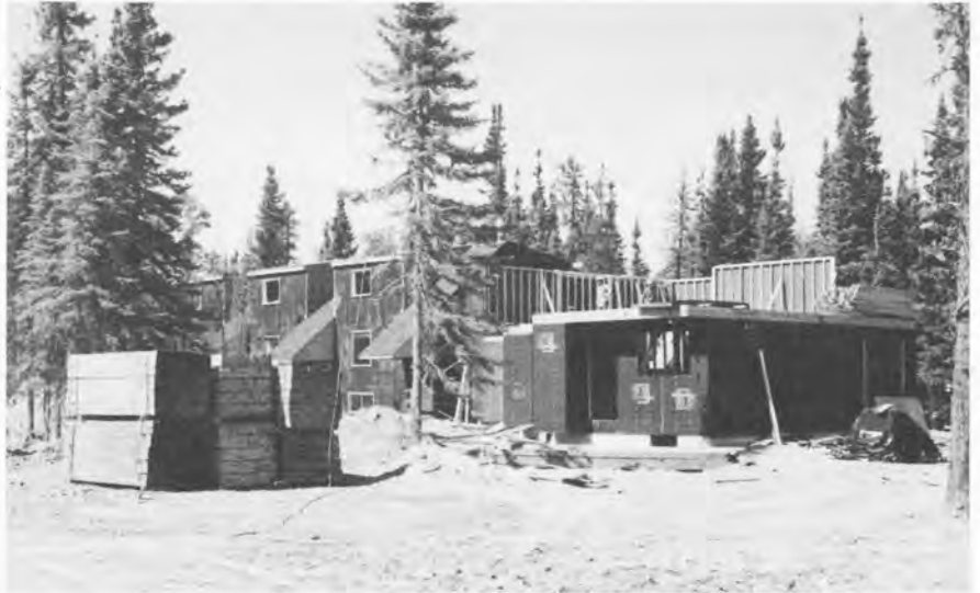
Townhouse under construction
