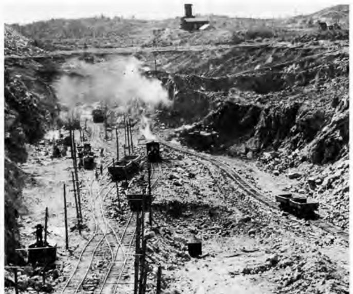
South end of open pit. The railway tracks were moved many times during the years of open pit mining. No. 2 shaft and shafthouse at top centre. (E. W. Gohl 1931)
