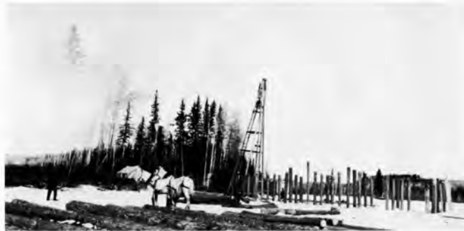
Piling for the Channing trestle was put in place during the winter months. Construction of the railway began in January 1928 and was completed by October 1928. (E. Germain 1928)
