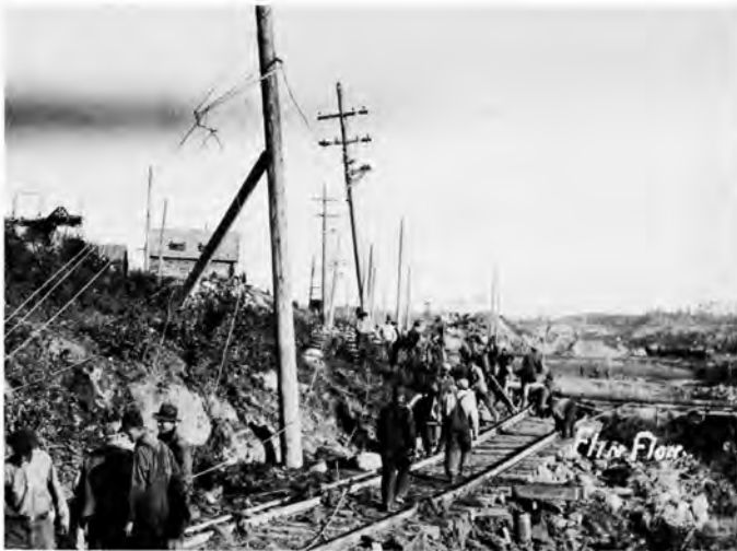
After blasting, railway tracks were laid for the electric locomotives. The old office perches on the edge of the pit. (H. Ennis 1931)
