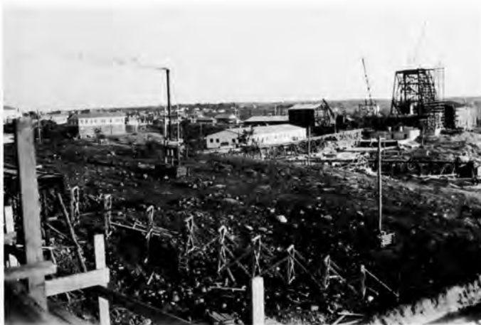
Head frame steel being erected. Mine changehouse in centre. (H. Ennis 1929)
