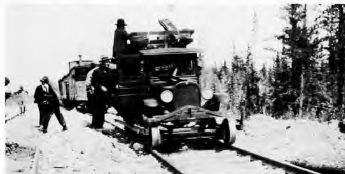
The Dominion Construction Company converted this car for easier transportation from one construction site to another. (F. A. Hollier 1928)
