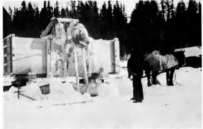
Seven of these wooden water tanks were used to ice the land stretches between the frozen lakes on the way to Island Falls. The ice covered land made travel much easier for the linn tractors and sleighs. (F. Willis 1928)
