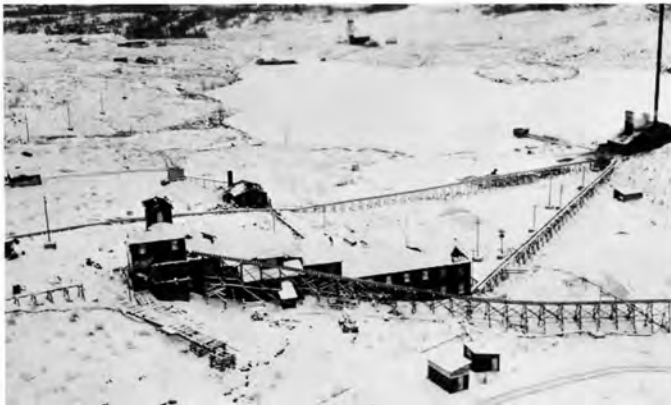
Construction of pilot mill began in August 1926 and went into operation March 1927. Steam lines ran from the powerhouse on the right to the assay office and mill. (H. Ennis 1928)
