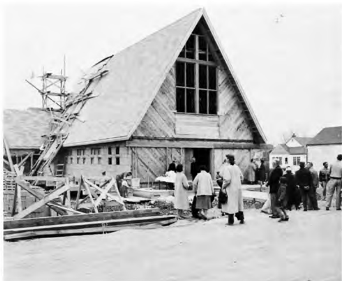
St. Paul's Catholic Church under construction, 1956. (Reminder)
