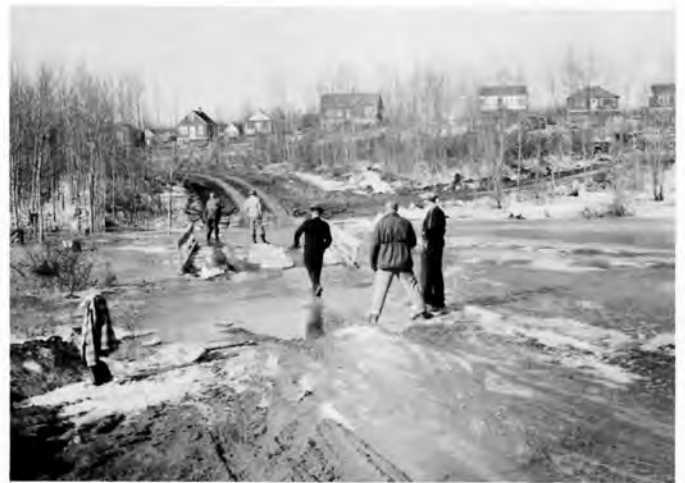
Lakeside bridge caused many problems, 1952. (Reminder)
