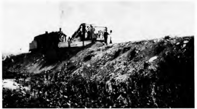
Rails were laid over frozen muskeg and gravel spread to prevent thawing under the tracks during warm weather. (F. Wells 1928)
