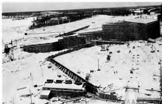
The mill steel almost completed. (H. Ennis 1929)
