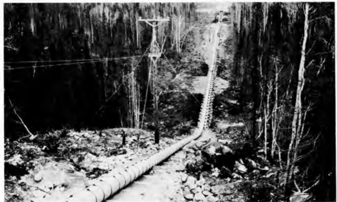
The twenty-inch wood stave pipe line ran from Cliff Lake to the company reservoir. (H. Ennis 1929)
