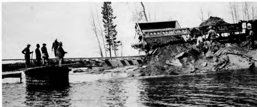
Building a reservoir at Flin Flon required some fill to build a dam. (HBM&S)
