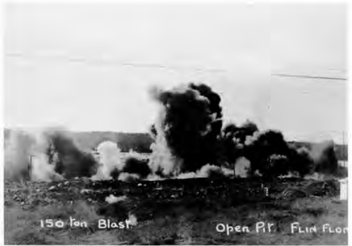
One of the largest blasts in the open pit was 150 tons of dynamite in 1931. Residents were warned prior to blast time and urged to remain in their homes. One story is told of rocks flying through a window and into a pot of potatoes. (Bea Halliday)
