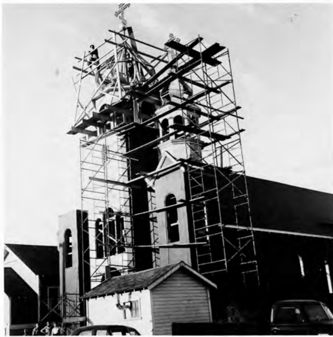
Scaffolding on St. George's Ukrainian Church, 1953. (Reminder)
