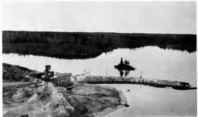
A dam was built across Flin Flon Lake to allow the water to be pumped out in preparation for excavation of the ore body by open pit mining. (W. S. B. Lockhart 1928)
