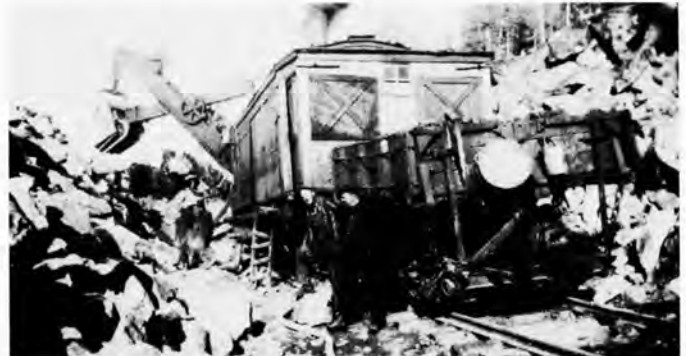
Clearing blasted rock. The side car was used for dumping gravel. (F. Wells 1928)
