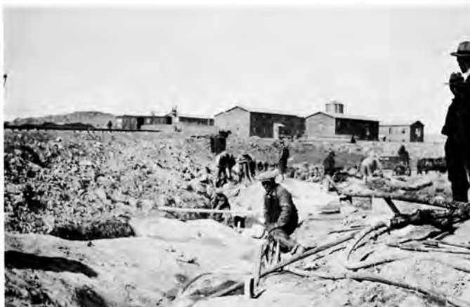
Drilling in preparation for blasting. Bunkhouses were built to house the construction workers. (H. Ennis 1929)
