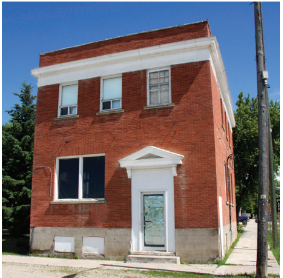
Brick bank building in Bowsman, 2014. It may soon be renovated into a Museum.
