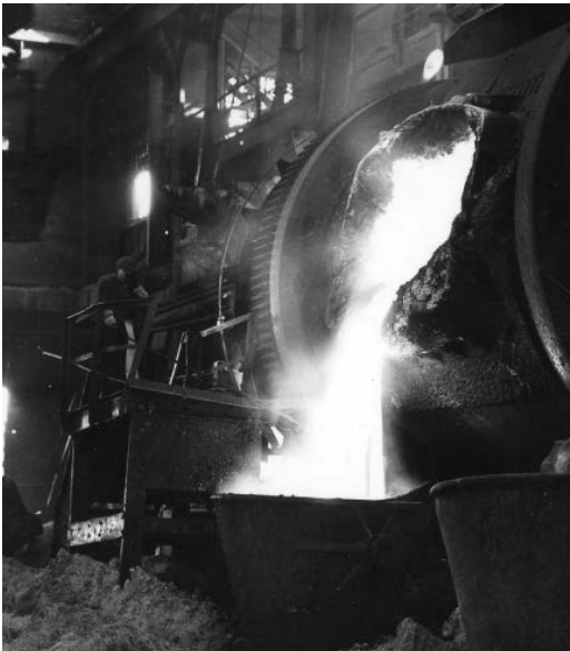
The converter furnace in the copper smelter, HBM&S.
