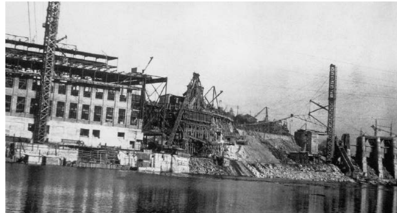
Construction at the Island Falls Powerhouse (left) and the Main Dam (right). 1929. (Flin Flon Community Archives)
