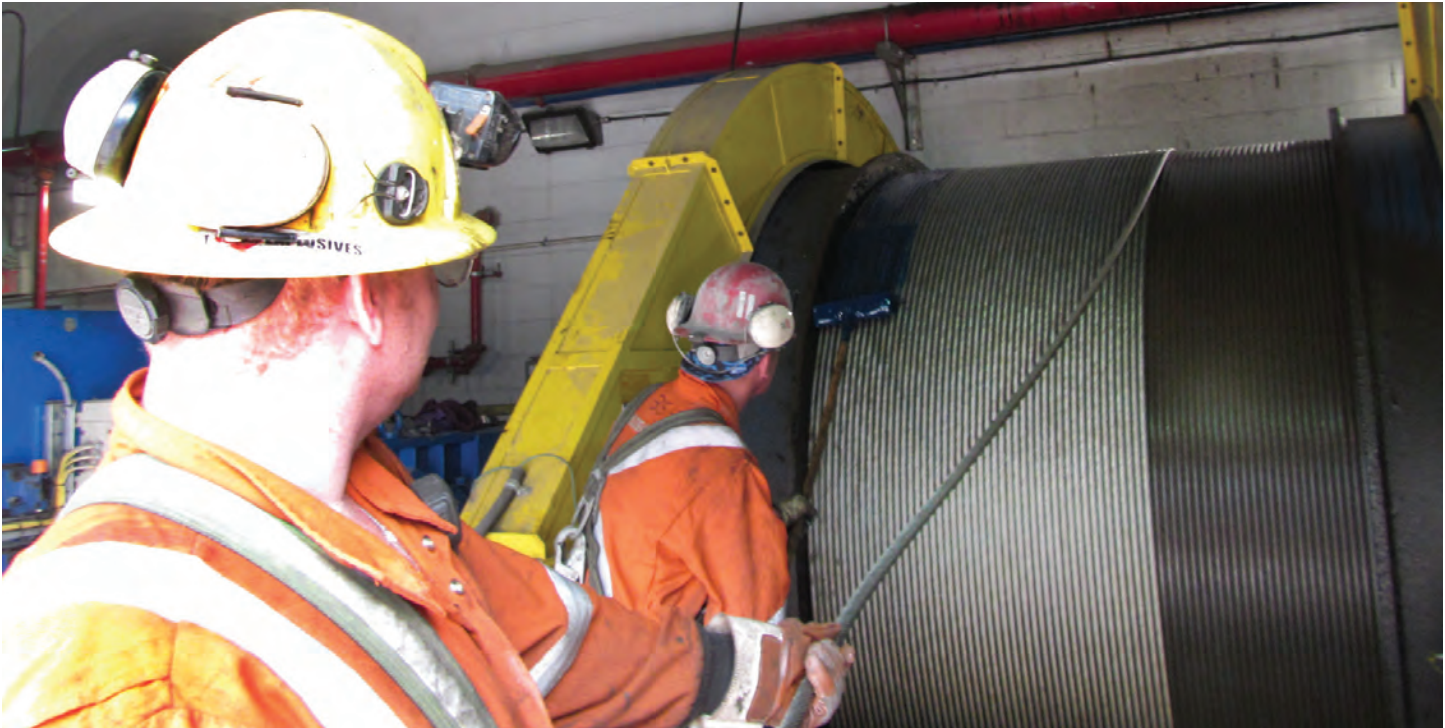
Jeremy Campbell (Shaft Inspector) and Seamus Lubinecki (Industrial Mechanic) ensure Lalor's new auxiliary cape rope goes on without a hitch. This was Lalor's first rope change.
