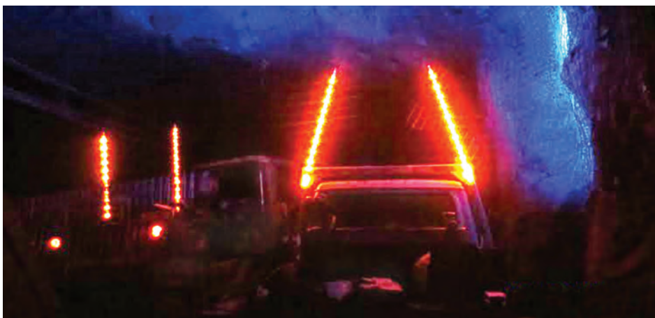
The new Safety lights added to the underground Toyotas.
